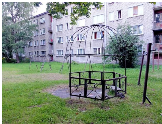
x - structure for recreation
