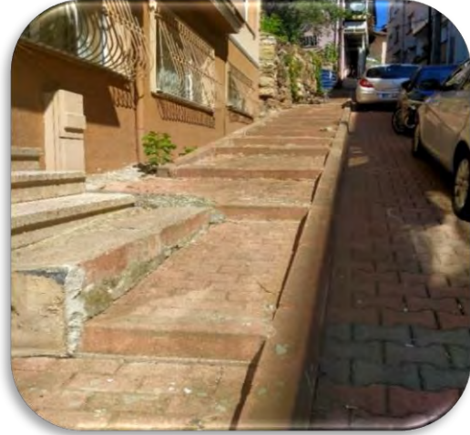
-Stairs on the side of the street
