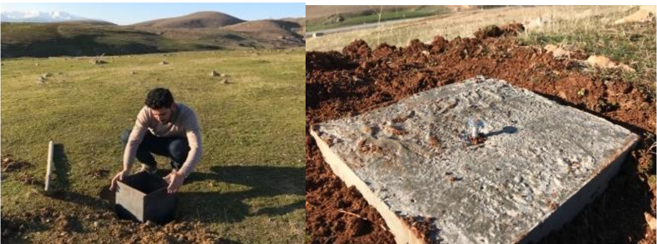
Figure 6: Establishment of Geodetic control points
