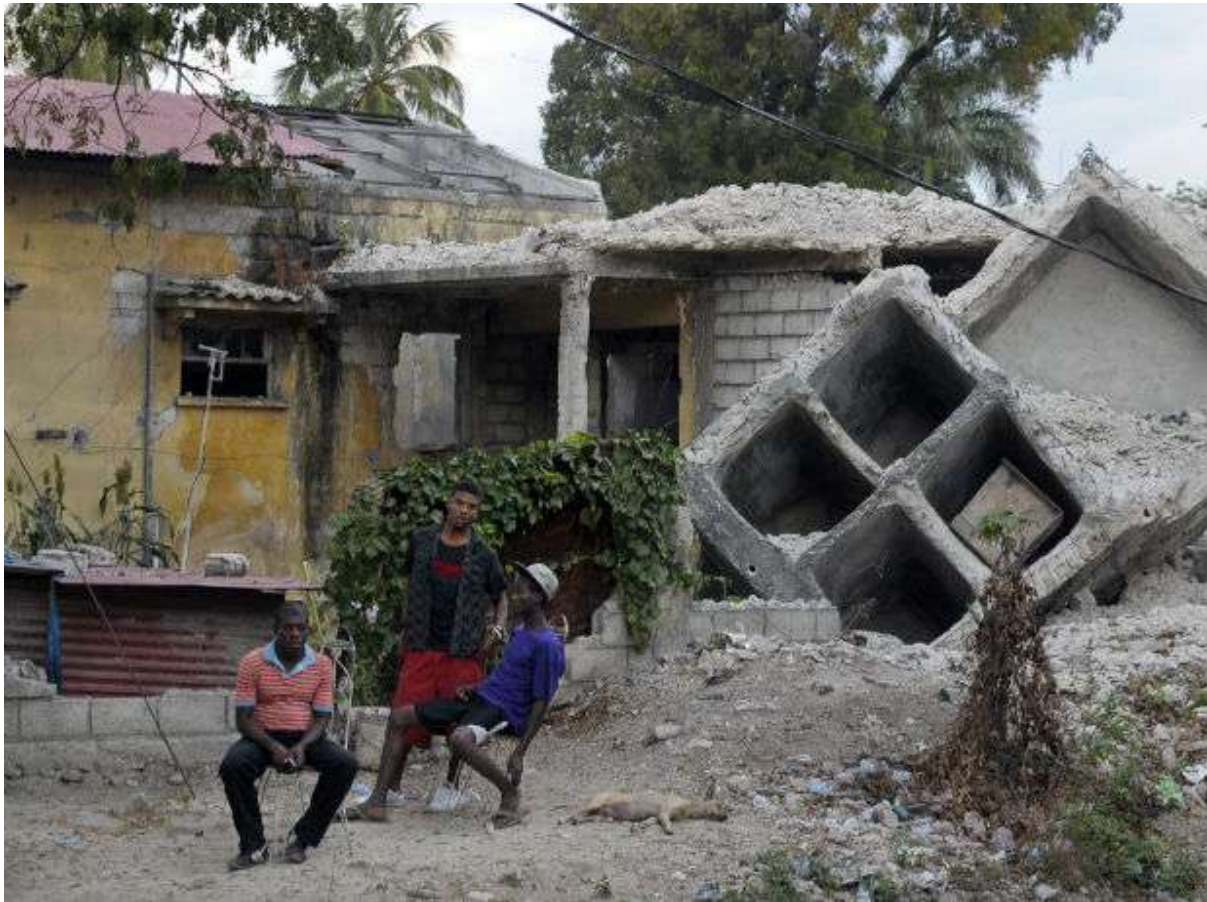
On January 4, 2012, people sit outside a house that was destroyed two years ago by the January 2010 earthquake in Port au Prince (Swoan Parker/Courtesy Reuters).
